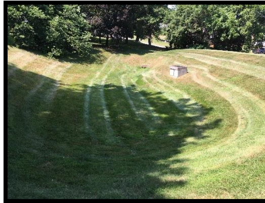
Figure 7: Overall View of Kilduff Circle Dry Extended Detention Basin
