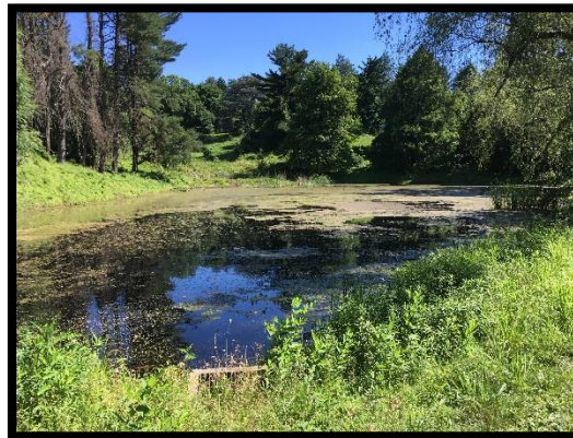
Figure 8: Overall View of Arborview Wet Pond
