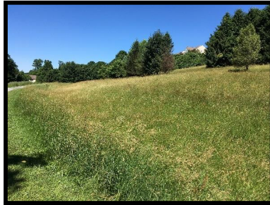
Figure 9: Overall View of Arborview Infiltration Trench
