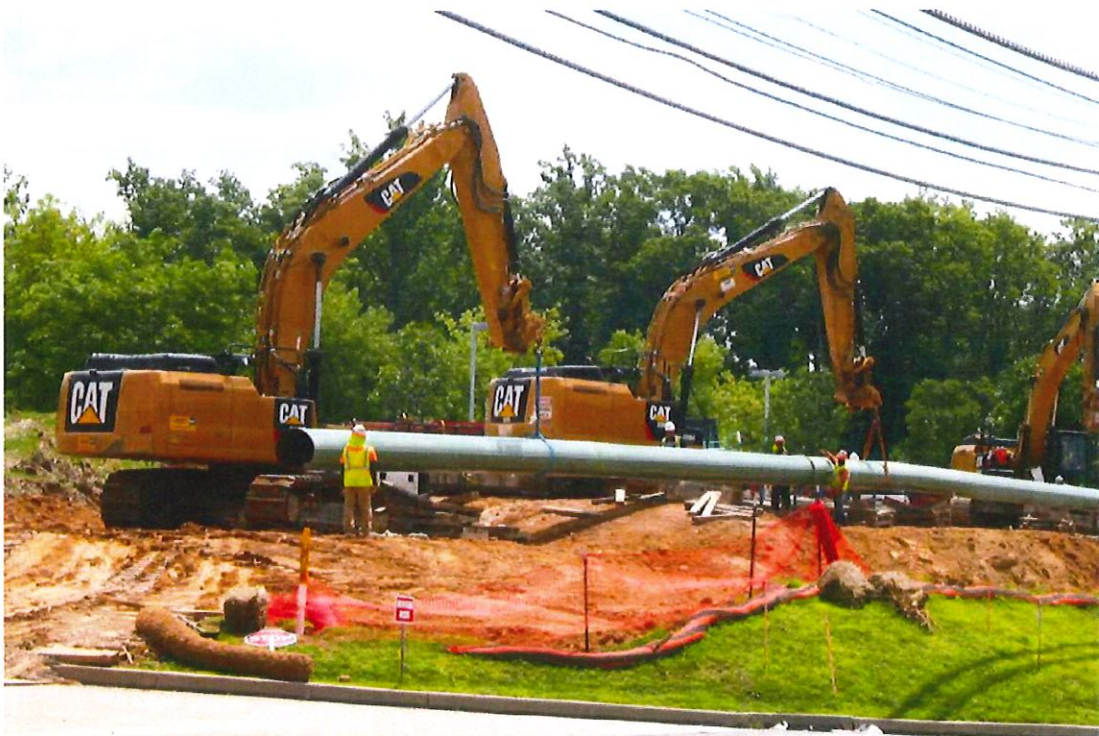
Better communication between stakeholders during the pipeline planning and construction phase could help reduce the impacts of pipeline projects on landowners, residents, and the environment.
