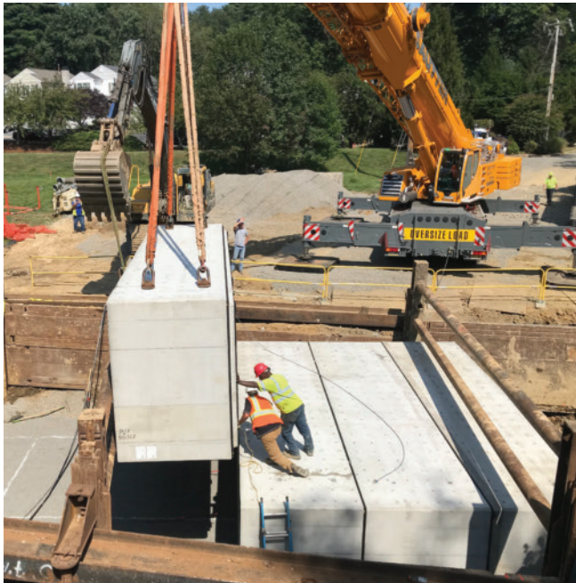
Oakbourne Bridge - Setting the Box Culvert
