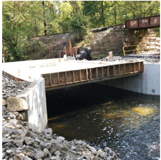
Oakbourne Bridge - Culvert Installation Complete
