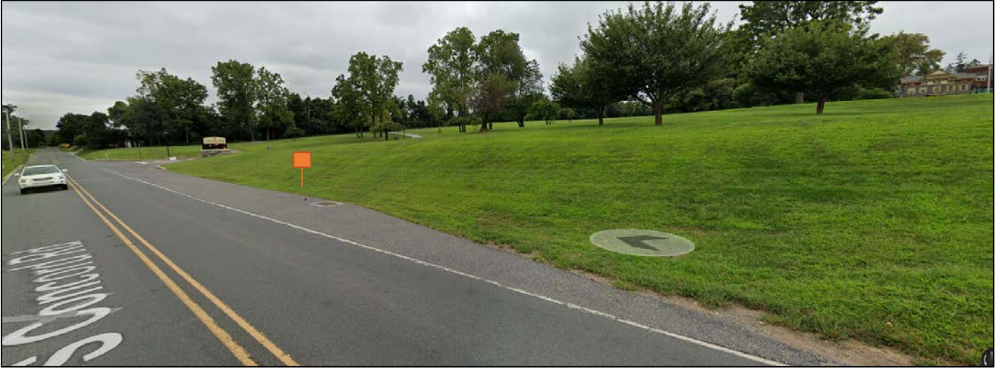
View from S Concord Rd heading south
