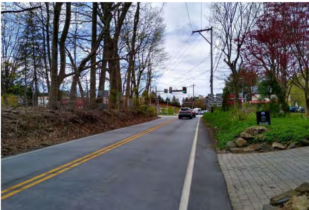
Westbound Street Road (SR 0926) looking west
