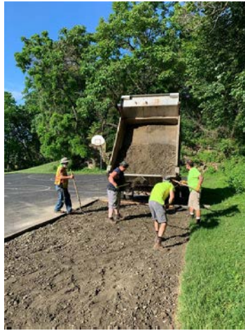
Basketball Court repair
