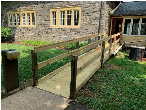
New accessible ramp at Oakbourne Mansion
