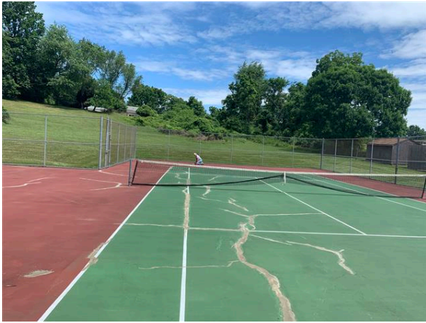
Tennis court repair
