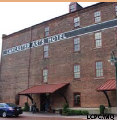
Warehouse to Hotel
