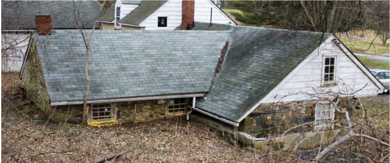
Original 1723 Hoopes building at Wynnorr Farm. Photo by Jim Guterl
