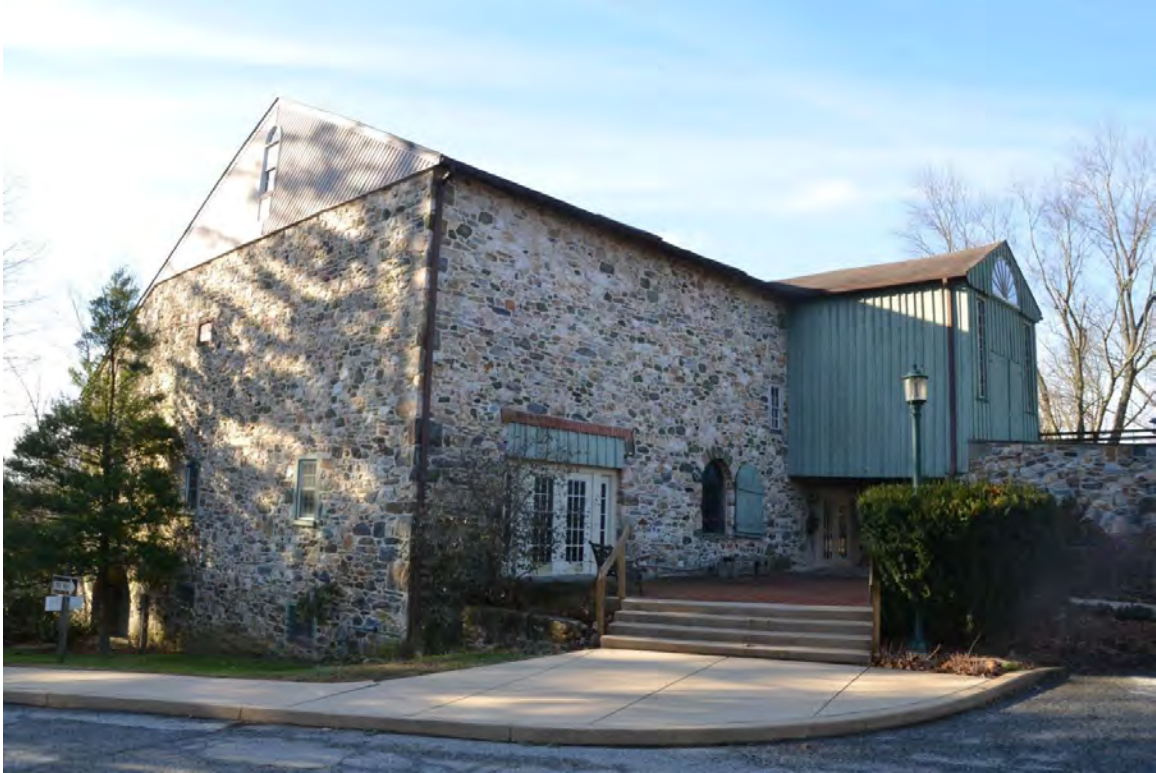
Osborne farm barn converted to worship space by Church of the Loving Shepherd. Photo by Jim Guterl.
