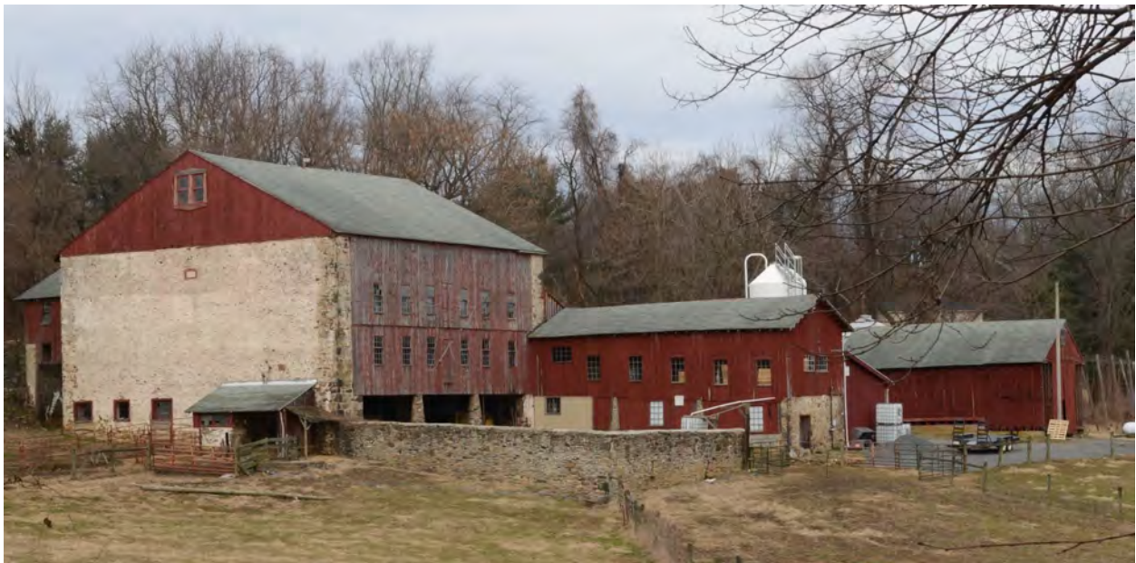
Wynnorr Farm barn with 1864 datestone. Photo by Jim Guterl
