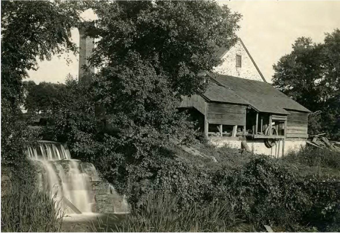
The large chimney in this 1895 photo indicates it was taken after a steam engine was added to the 1839 sawmill. This was added to the 1801 gristmill (the stone building). The steam engine, most likely in the corner of the mill, was replaced with water power in 1895. Photo courtesy Westtown School Archives.
