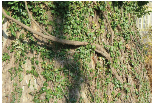
Details of the vine stems on the London Plane's trunk which were cut and removed
