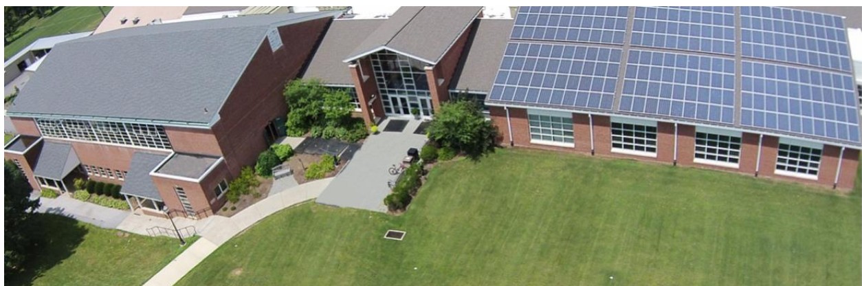
Solar PV on Westtown School Athletic Center
