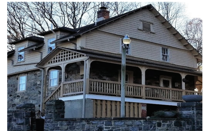
The Oakbourne Park gatehouse/tenant house, formerly Jesse Mercer's schoolhouse, c. 1807. The stone section is likely part of the original school.
