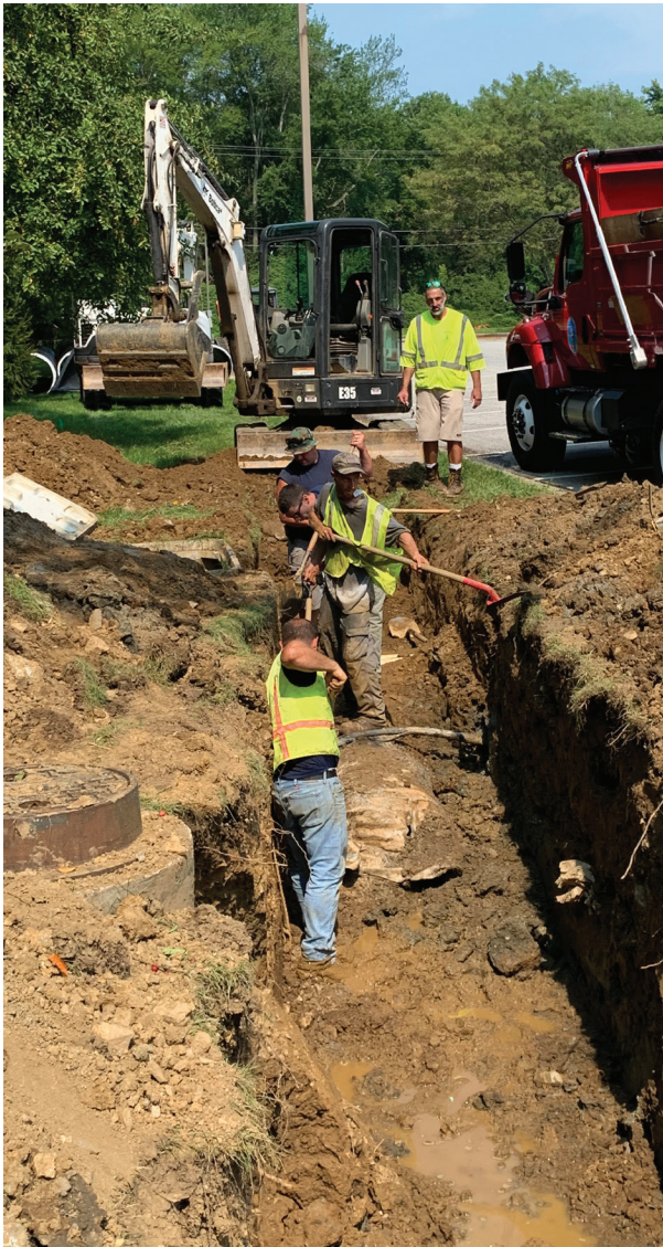
During Tropical Storm Isaias, a stormwater pipe near the Kirwood Business complex off Green Lane collapsed. Public Works replaced 160' of stormwater pipe, dodging underlying sewer, water, and telecommunication lines.
