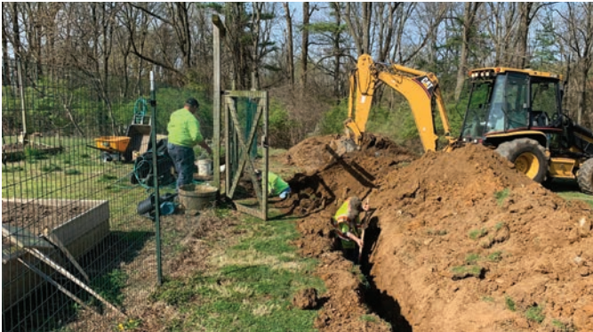
At Oakbourne Park, the crew demonstrated their prowess with both machines and hand tools when they installed water service to the Community Garden, so the gardeners no longer have to run a long hose from the Oakbourne Pavilion. The ramp into the mansion was also replaced this summer.
