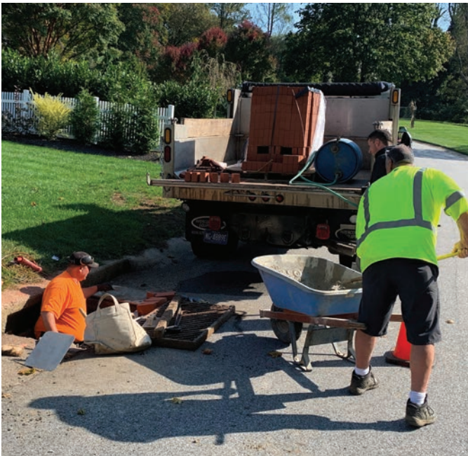
Reconstruction of a stormwater inlet.
