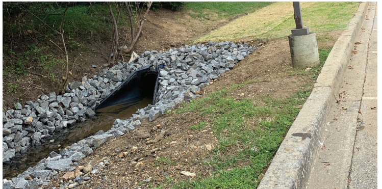
During Tropical Storm Isaias, a stormwater pipe near the Kirwood Business complex off Green Lane collapsed. Public Works replaced 160' of stormwater pipe, dodging underlying sewer, water, and telecommunication lines.
