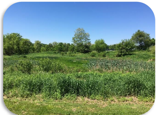
Constructed wetlands at Bayard Rustin High School, 2018
