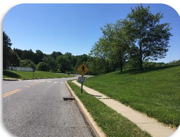
Sidewalk along Skiles Blvd., 2018
