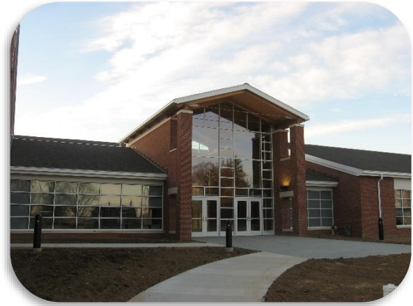
Environmentally-friendly athletic center at Westtown School was completed in 2007.
