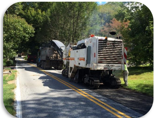
Milling on Little Shiloh Rd, 2014
