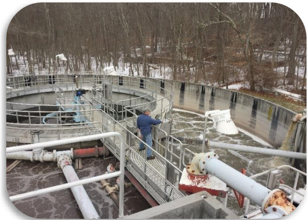
Westtown-Chester Creek Wastewater Treatment Plant, 2015
