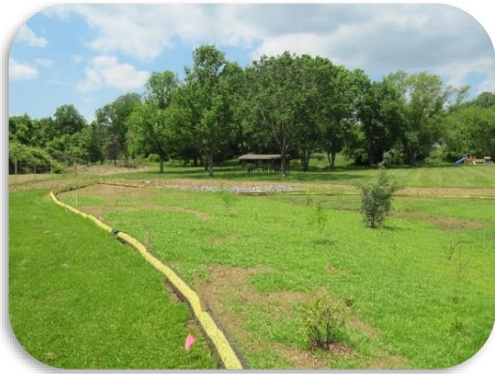
Bioswale at Tyson Park, 2015
