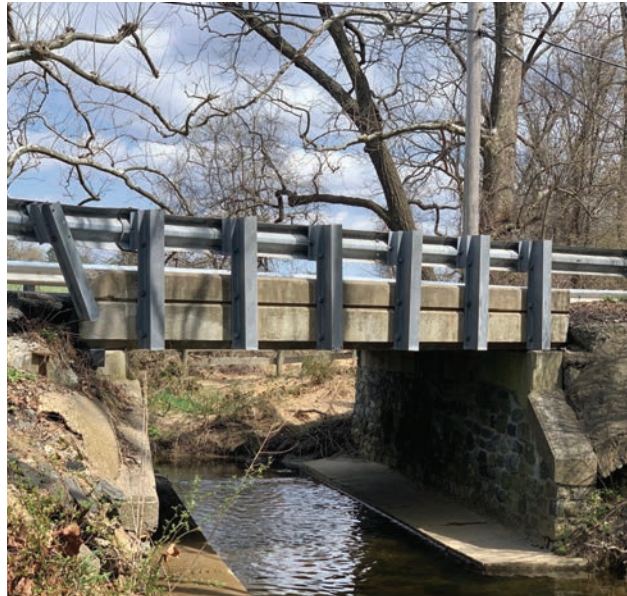
S. New Street Bridge over Radley Run
