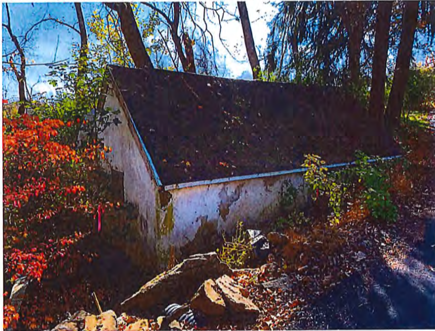
Photograph of the existing spring house located on site. View is of the north side of the spring house, looking south.
