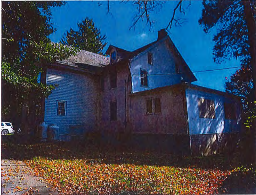
Photograph of the existing farmhouse located on site. View is of the northwest corner of the dwelling, looking southeast.
