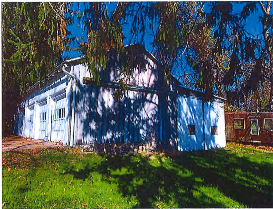
Photograph of the existing detached garage located on site. View is of the east side of the garage, looking west.
