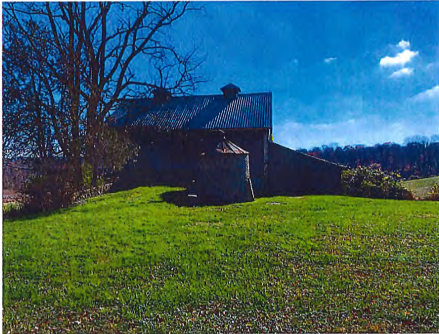
Photograph of the existing barn located on site. View is of the north side of the barn, looking south.
