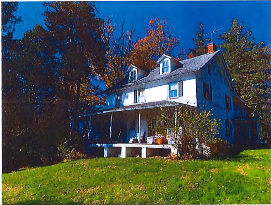
Photograph of the existing farmhouse located on site. View is of the south side of the dwelling, looking north.
