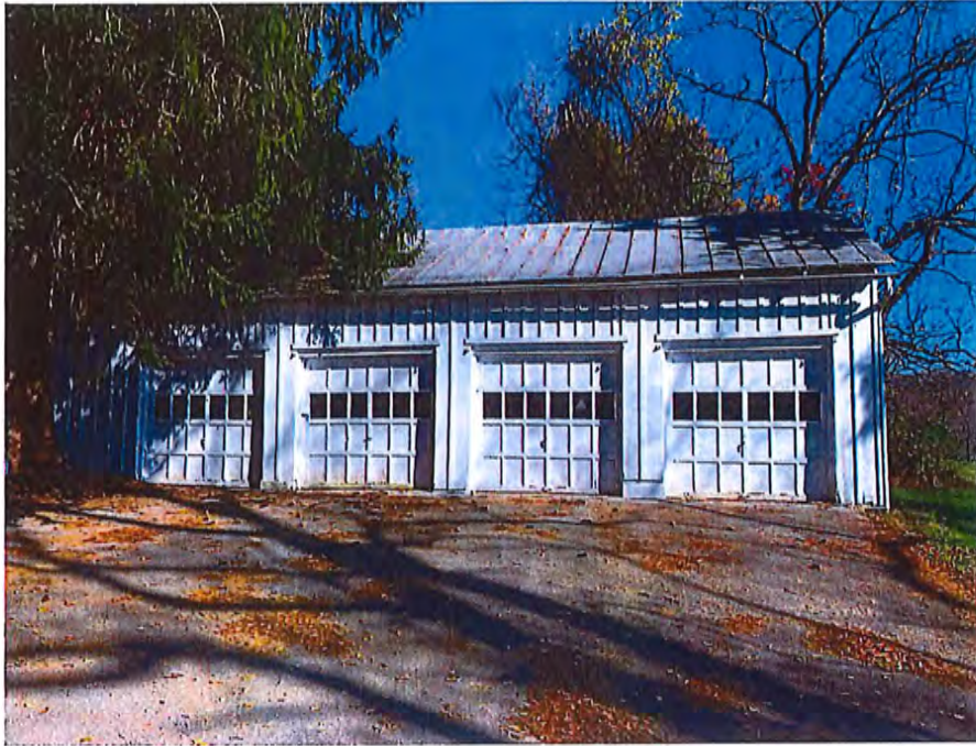
Photograph of the existing detached garage located on site. View is of the south side of the garage, looking north.
