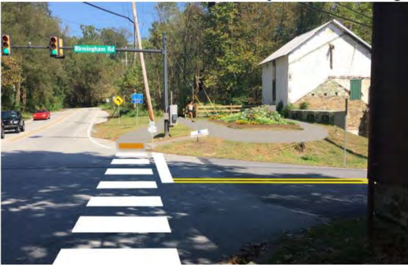
Figure 3.3: View south along Birmingham Road (40 MPH)
