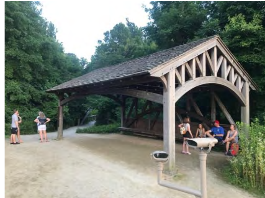
Standalone covered pole barn
