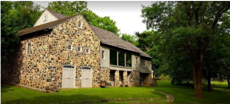
Barn Visitors Center
