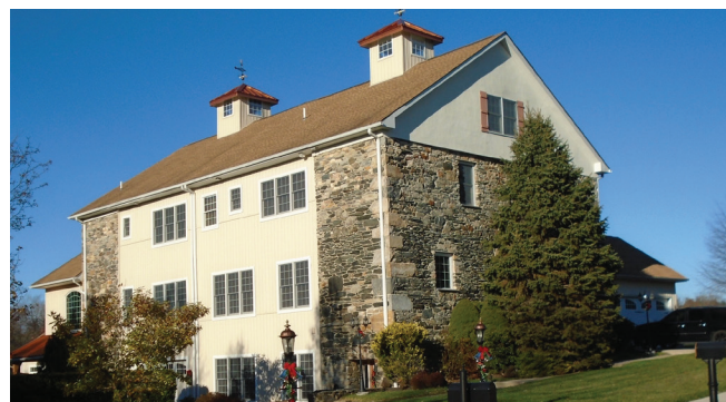
The Cherry Creek Barn was retained and renovated into 2 residences in a technique known as adaptive reuse
