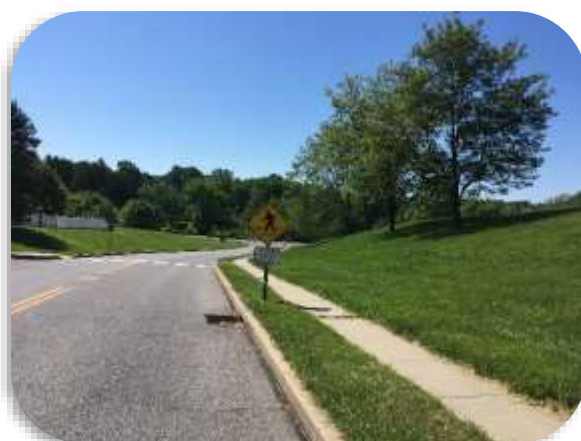
Sidewalk along Skiles Blvd., 2018
