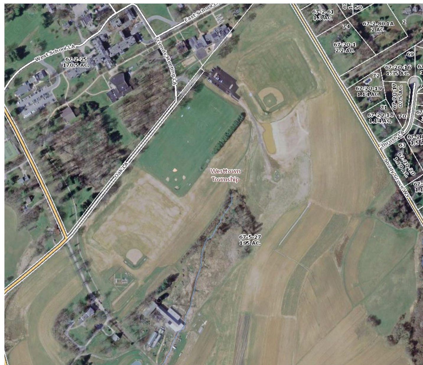
This 2005 aerial image depicts the recent construction of the present-day Varsity Baseball and Softball fields as well as an expanded multi-purpose field area between the Softball and Junior High Baseball fields. Fill material generated during the construction of the Varsity Baseball field was used to flatten the area where the Softball and expanded multi-purpose fields are shown. The resultant man-made steep slopes at the southwest corner of the fields are visible in dark green. [9]
