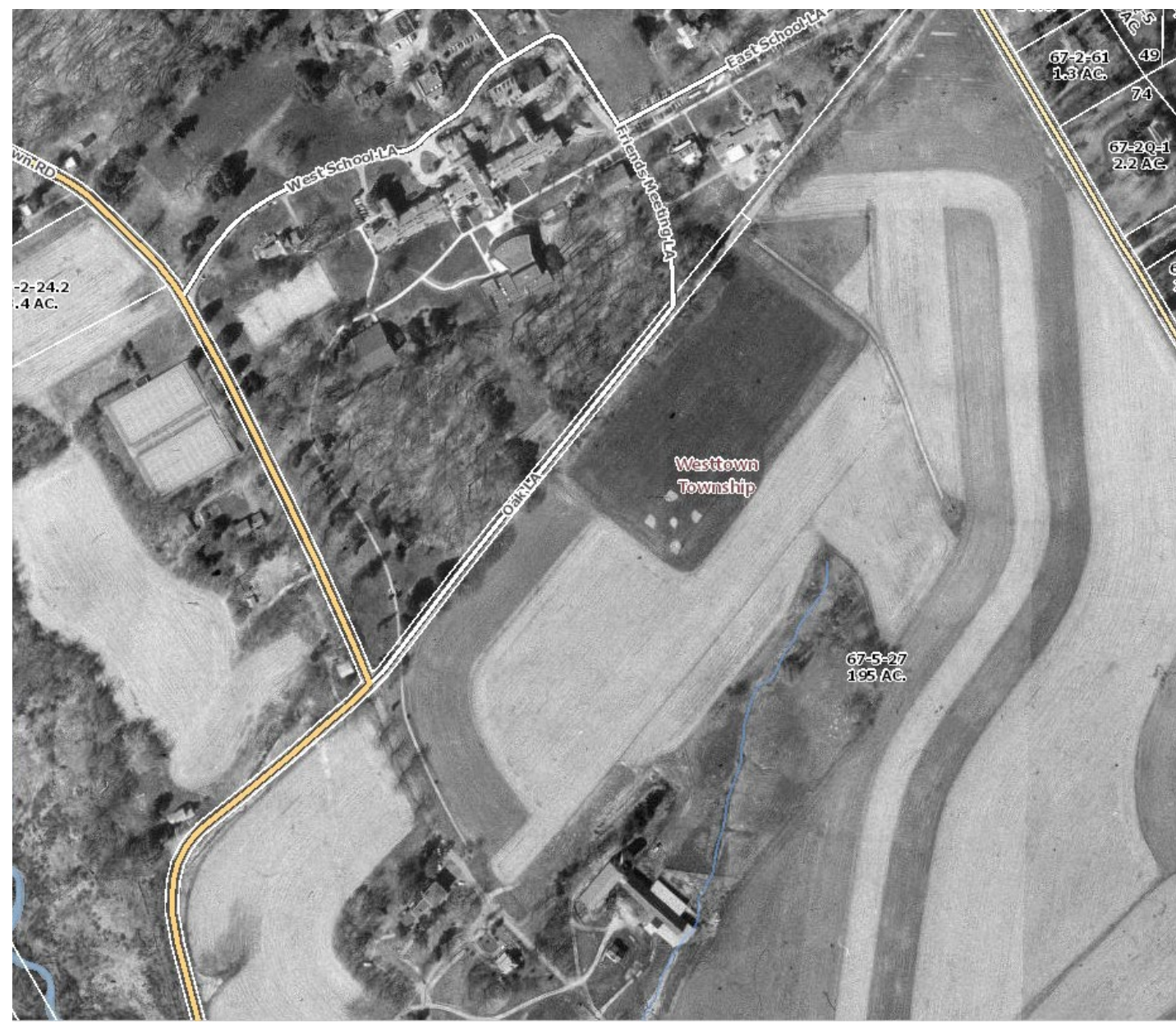
1993 satellite image depicting the location of Westtown School's Junior High Baseball field with overlay/ multi-purpose fields visible to the northeast. The present-day Varsity Baseball and Softball fields have not yet been constructed. The area where the synthetic turf fields are proposed remains in agricultural use. [7]
