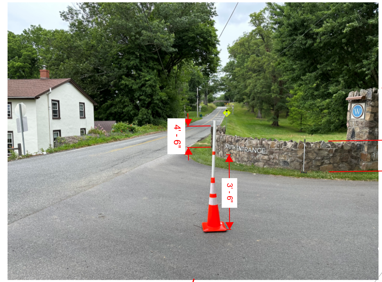
Oak Lane Approach Looking to the Right
