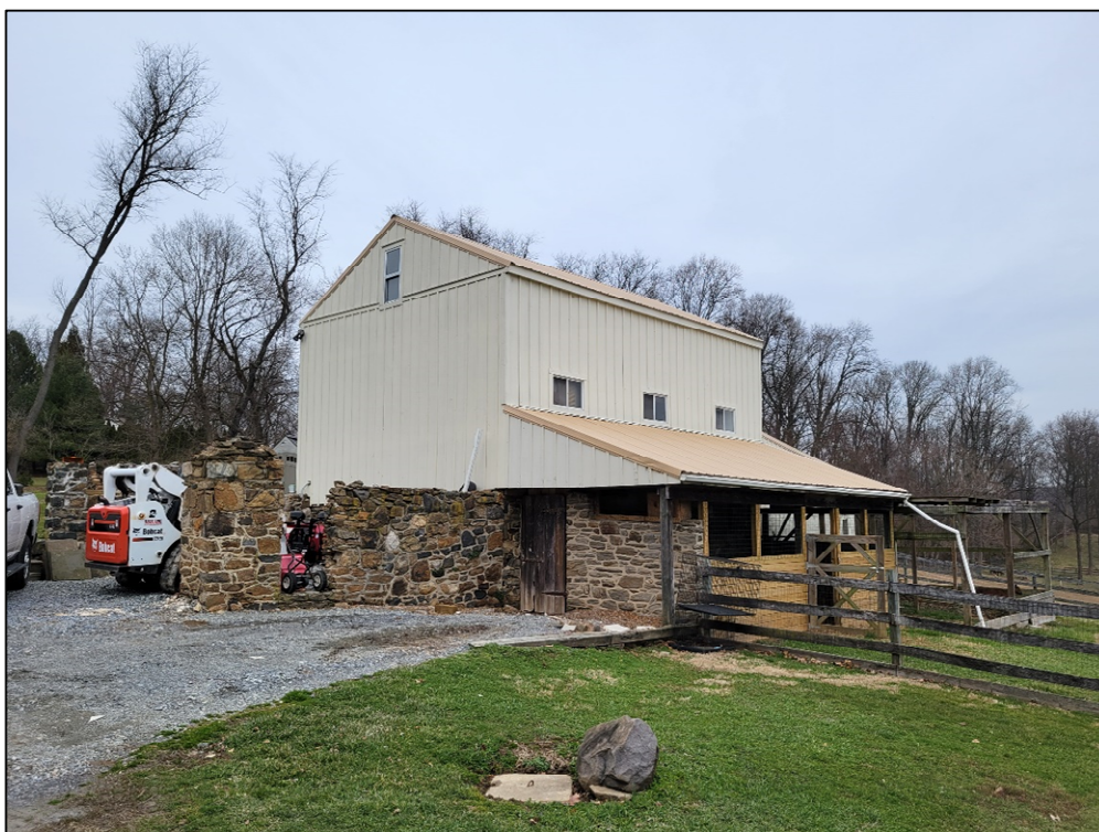
Photo 6. Barn, facing north. The stone foundation on the left may have been the foundation of a now-lost Speakman woodworking shop.
