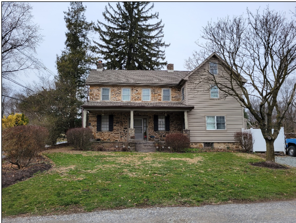
Photo 2. Main elevation of the Miles House, facing northwest, showing the stone core on the left and the 1879 frame addition on the right.
