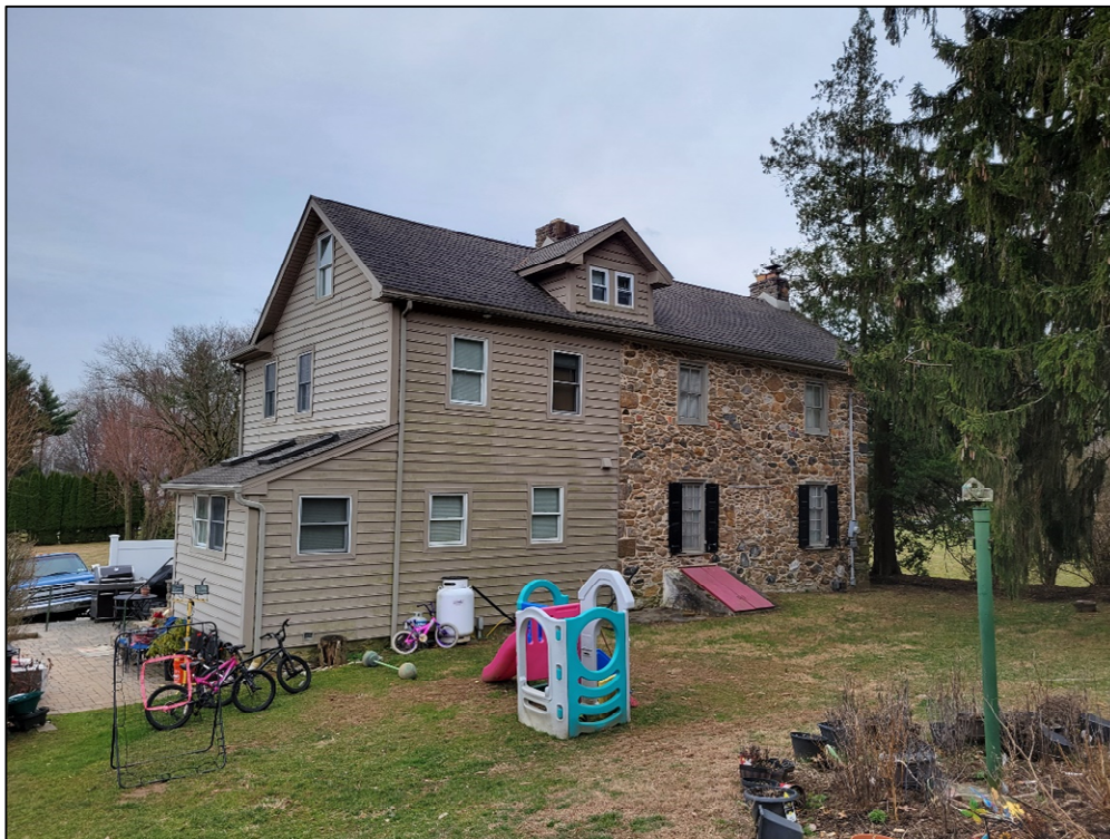
Photo 5. Rear of the Miles House, facing south, showing the three sections (small addition, 1879 frame addition, and stone core).
