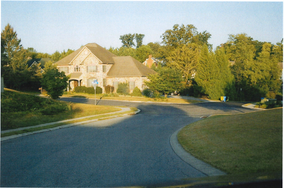
Ashleigh Drive (10.4% grade) with horizontal and vertical curvature on the roadway
