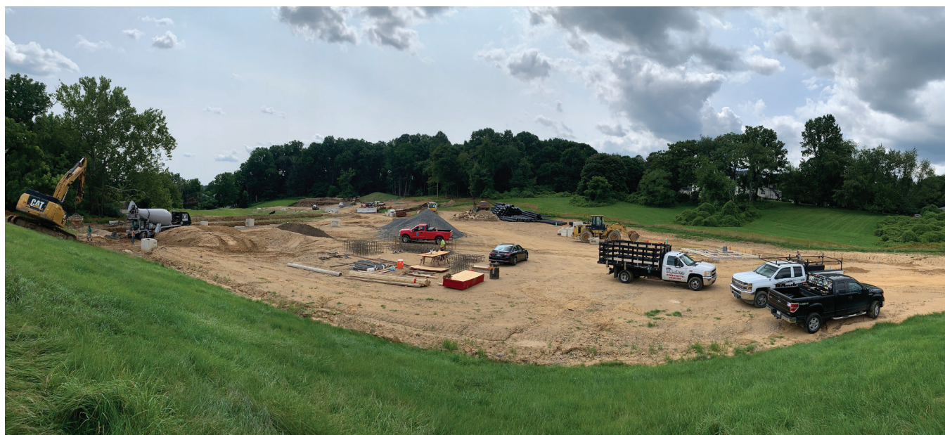
Oakbourne Park Athletic Complex site preparation
