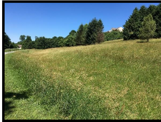
Figure 9: Overall View of Arborview Infiltration Trench
