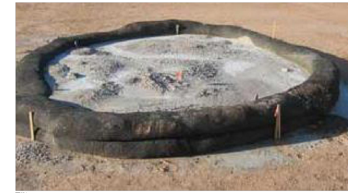
FIGURE 3.18 Typical Compost Sock Washout Installation
