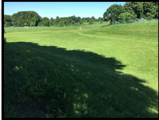
Figure 10: Overall View of Stetson Middle School Dry Extended Detention Basin
