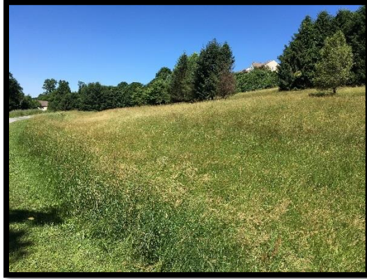
Figure 9: Overall View of Arborview Infiltration Trench
