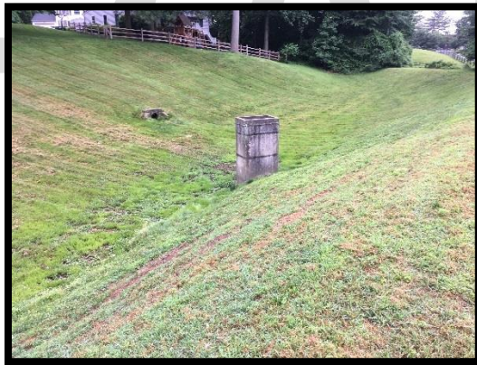
Figure 6: Overall View of West Glen Dry Extended Detention Basin
