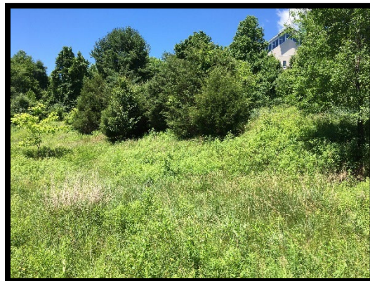
Figure 4: Overall View of Simon and Jude Dry Extended Detention Basin
