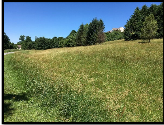
Figure 9: Overall View of Arborview Infiltration Trench
