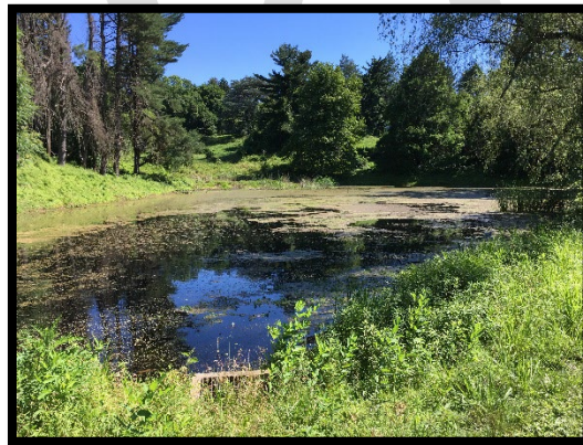
Figure 8: Overall View of Arborview Wet Pond
