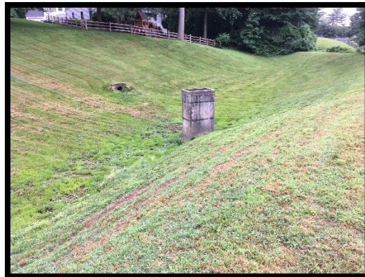
Figure 6: Overall View of West Glen Dry Extended Detention Basin
