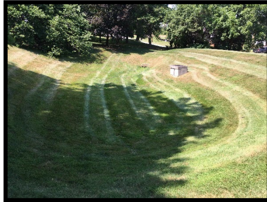
Figure 7: Overall View of Kilduff Circle Dry Extended Detention Basin
