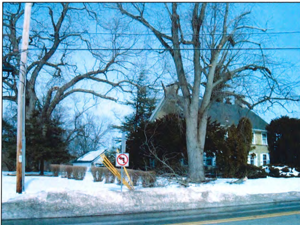
Photo 2 – West and south elevations of Westtown Inn, looking northeast
