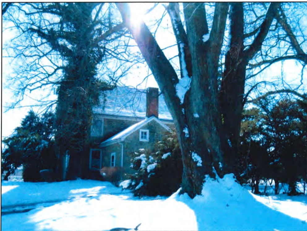
Photo 11 – North elevation of Westtown Inn, looking south
