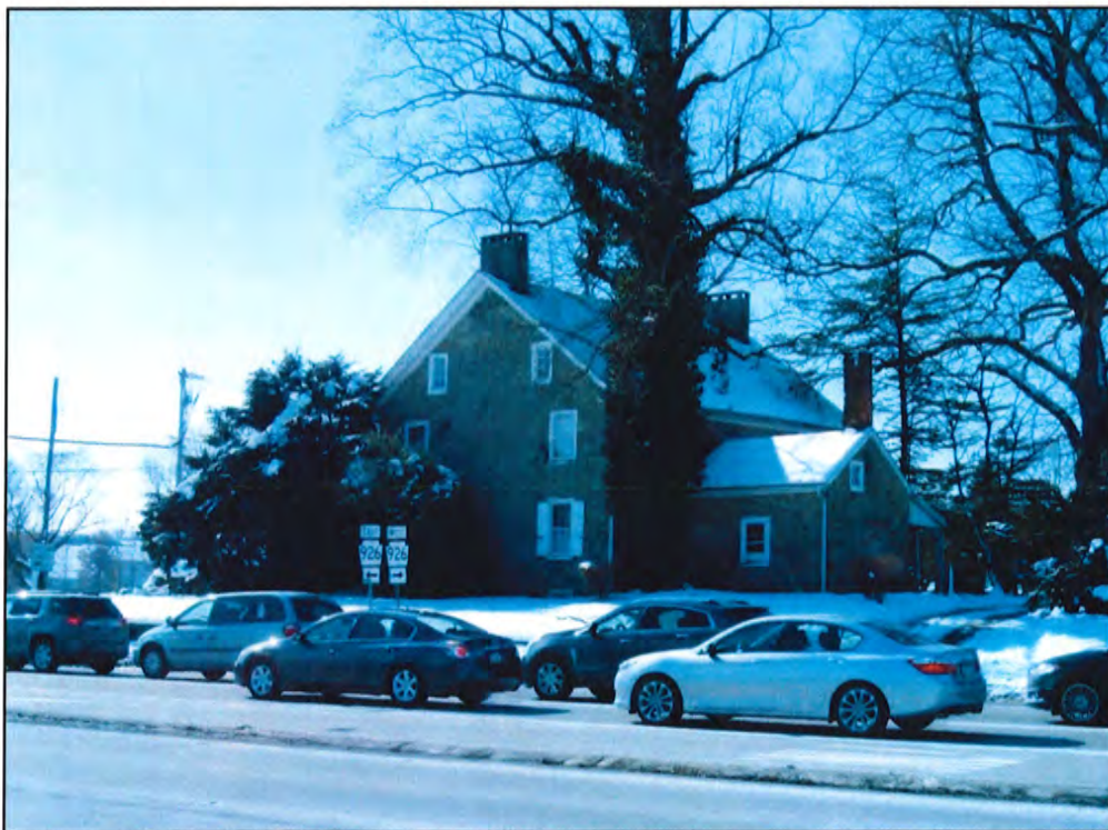
Photo 9 – East and north elevations of Westtown Inn, looking southwest
