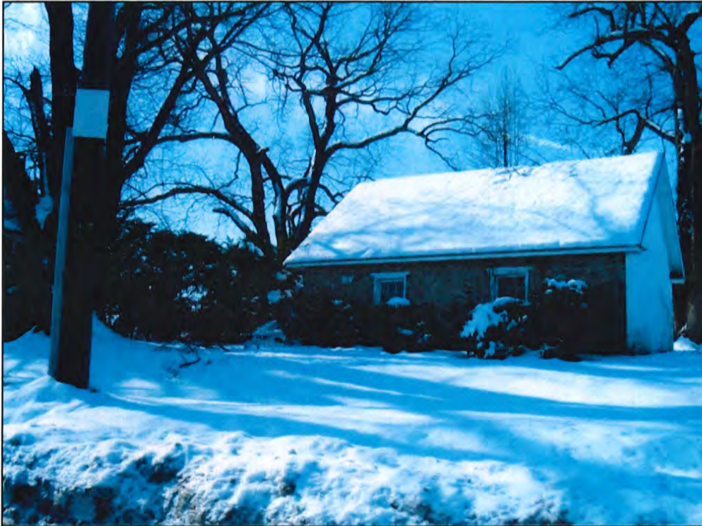
Photo 14 – East and north elevations of garage at Westtown Inn, looking southwest
