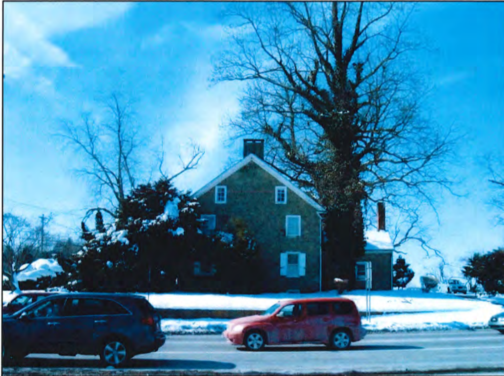
Photo 6 – East elevation of Westtown Inn, looking west
