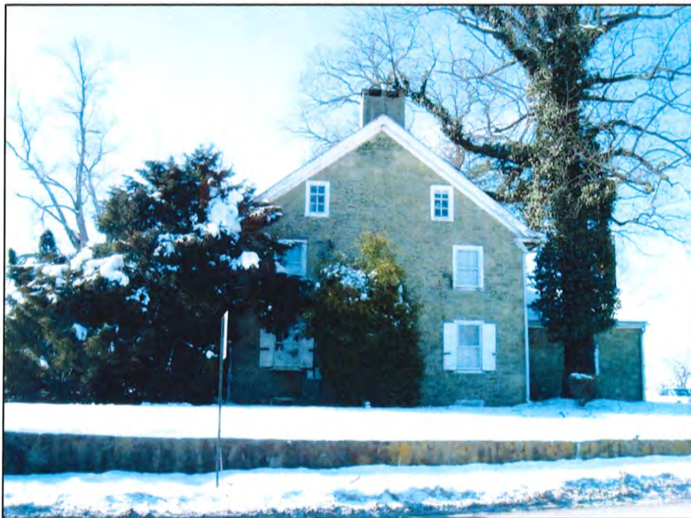
Photo 7 – East elevation of Westtown Inn, looking west
