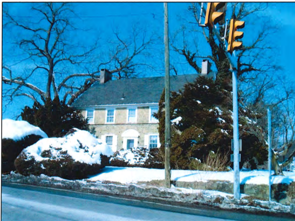
Photo 4 – South elevation of house looking northwest
