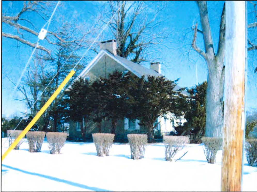
Photo 12 – West elevation of Westtown Inn, looking northeast
