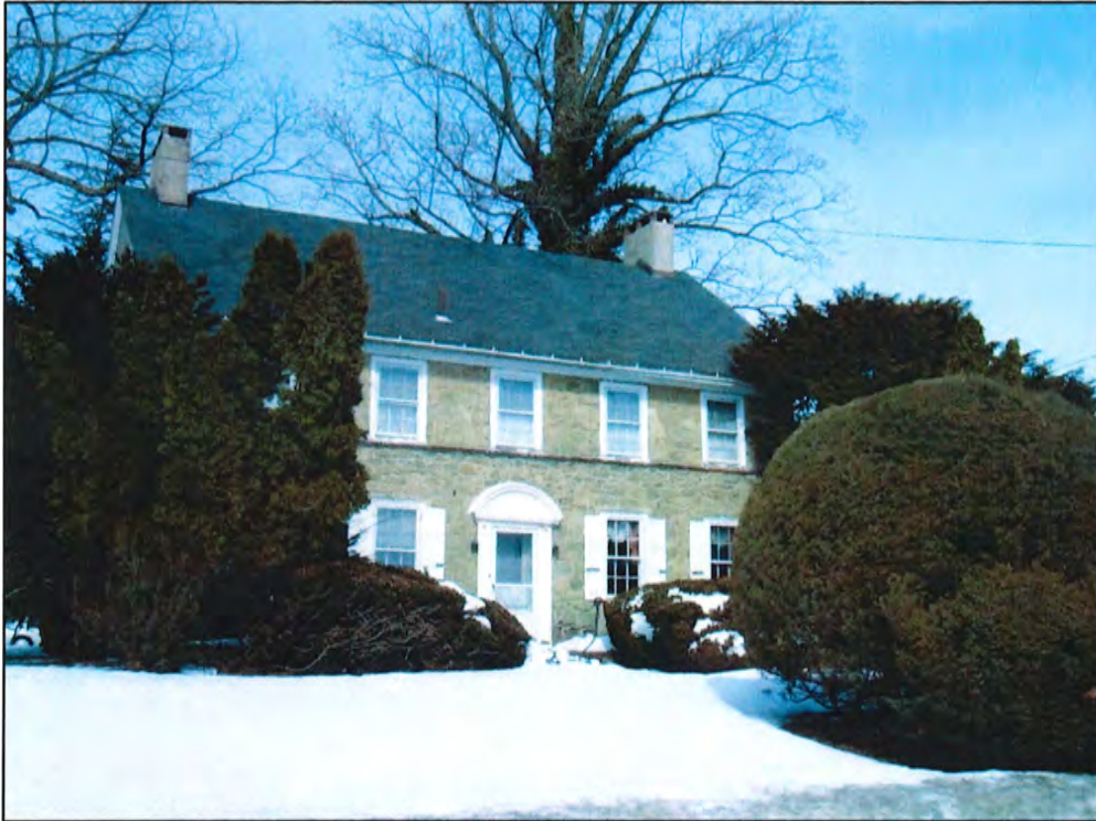
Photo 3 – South elevation of Westtown Inn, looking north
