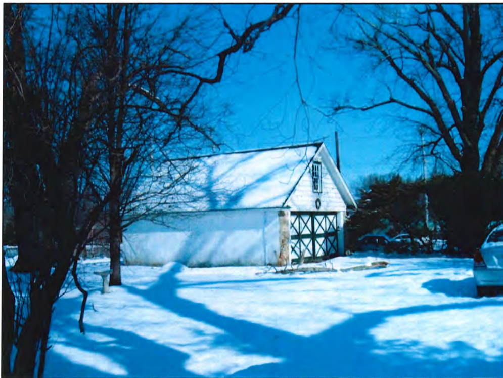
Photo 13 – West and south elevations of garage at Westtown Inn, looking northeast
